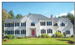
GULFORD $874,900 - Magnificent custom col on a cul-de-sac 1.5 miles to town impressive LR w/columns to FRM w/open flr plan beautiful arches to state of the art kitchen w/cherry cabinets & granite counters & ctr island dr w/9' ceilings sep staircase to bonus room w/fpl. Sue Clifford and Patty Gallagher 203-245-4700, VM206 or VM210.
